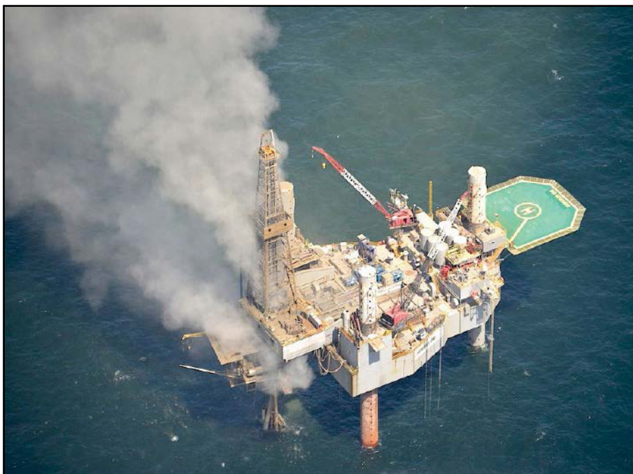
Fig. 1. The Hercules platform in flames on 23 July 2013.
